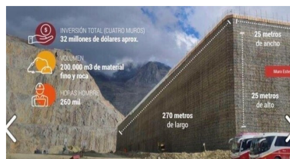
Figure 4: Final as-built design, including a mechanically stabilized earth (MSE) wall optimized through the integration of RACS, designed for a 70 kPa impact pressure and commissioned in 2021.
