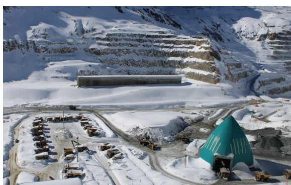
Figure 5: Mechanically stabilized earth avalanche dam providing permanent protection for the primary crusher against avalanche impacts.
