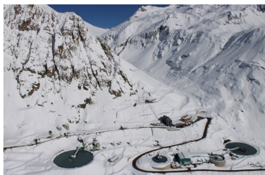
Figure 7: Access to the concentrator plant, located in a high-avalanche-exposure sector.
