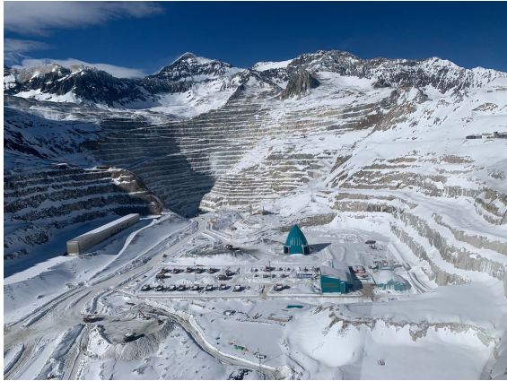
Figure 3: Overview from the strategic operational NODO 3500 sector where the main crusher of the open pit is located. On the left side the catching dam 25 meter height and width and 270 meter long protecting the East side of the area.
